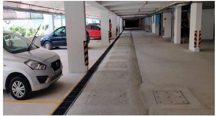
Figure 38 : Eco-STP under cafeteria & Parking
